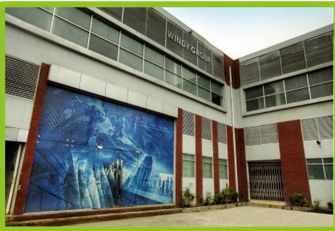
Windy Wet & Dry Process Ltd. U-2.
