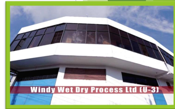
Windy Wet & Dry Process Ltd. U-3.
